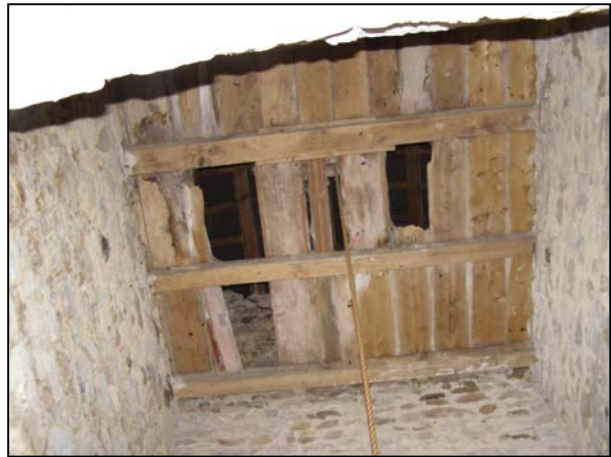
Looking up inside the Bell Tower ↑
